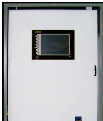
Panel insert front view – all you see is the MIDAS HMI touch screen
