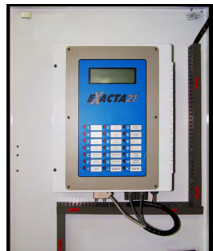
Panel insert back view – EXACTA21 keypad acting as a "hot back up" to the MIDAS
